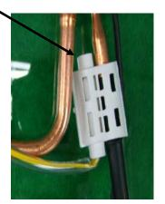
The Sensor mounted correctly.
